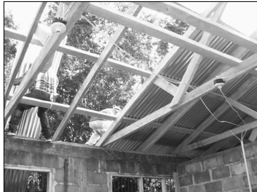
Looking up at the Maintenance Roof Construction.
